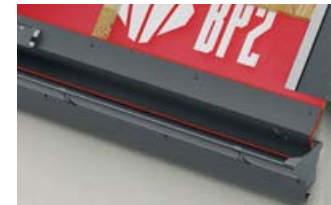
Starting drip-edge flashing for the gutter
